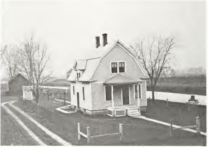
Patrolman's house on the feeder, 3.9 miles north of the summit. (Photograph courtesy of Hennepin Canal Parkway.)
